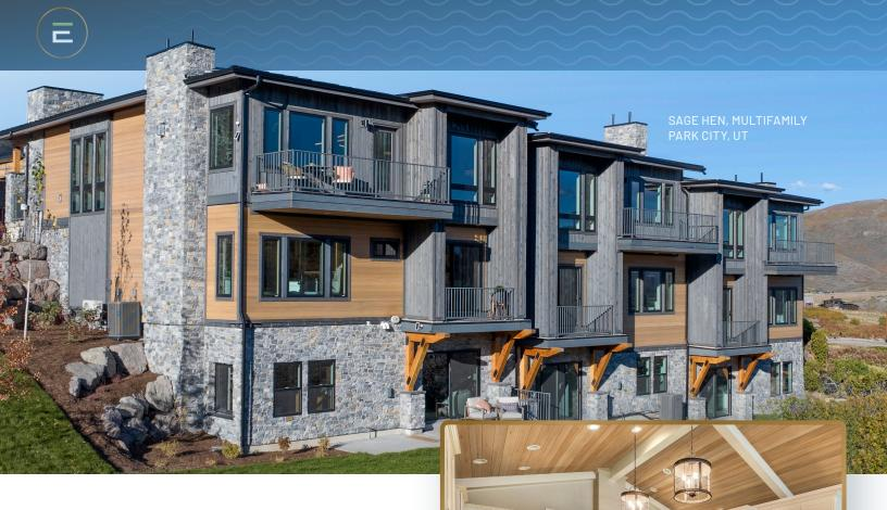
The thermal modification process stabilizes the wood with heat and pressure and makes it highly resistant to rot, shrinking and seasonal shifts, creating an exceptionally durable board. This process darkens the wood and natural mineral streaks may occur.
