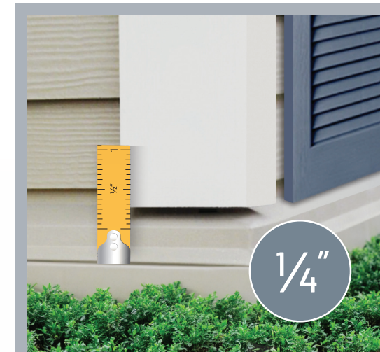
At least 1/4" above brick, concrete or flashing to allow for water drainage.
